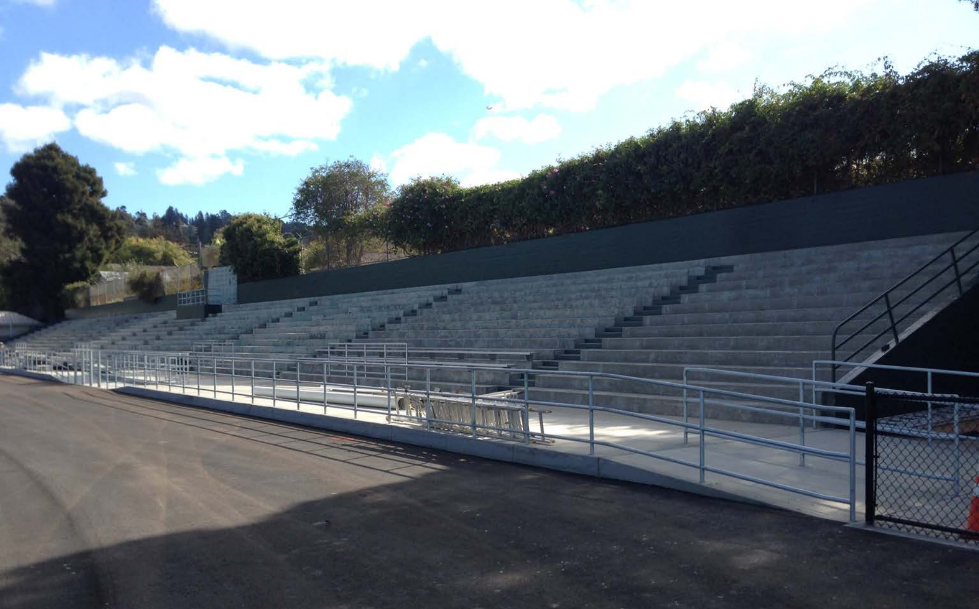
10.c. El Cerrito High School Stadium Bleachers
